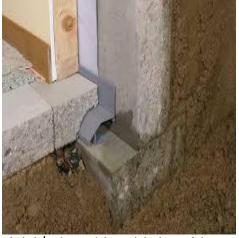
Above are examples of foundation interior wall drainage. Note that <u>ALL of the edges and seams are sealed air/moisture tight</u>, and the <u>base of the</u> <u>membrane drains into a drain system</u>. THIS IS THE MOST EFFECTIVE WAY OF PREVENTING MOISTURE *(and RADON)* ENTRY INTO THE BASEMENT. IF ANY FORM OF FINISH IS INSTALLED IN BASEMENTS, THIS IS THE PREFERRED METHOD OF PROTECTION IN MY OPINION. *(images are examples from web)*
